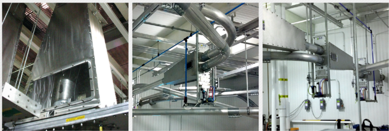
8" (203mm) Flex Tube Diverter handling PVC compound
